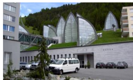
The completed green roof.
