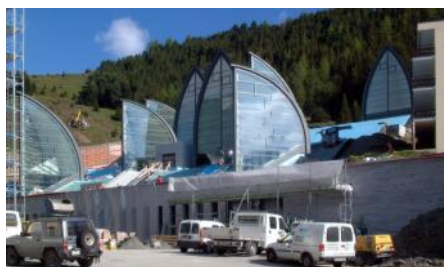
Installing the thermal insulation layer above the roof waterproofing.
