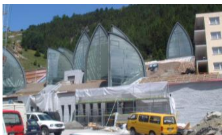
Fitting the wooden construction that resembles an "avalanche support".
