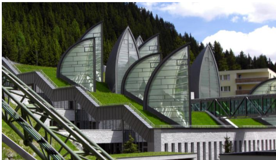
The eight light sails – a construction made of steel and glass.
